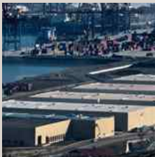
Storage and distribuion zone
